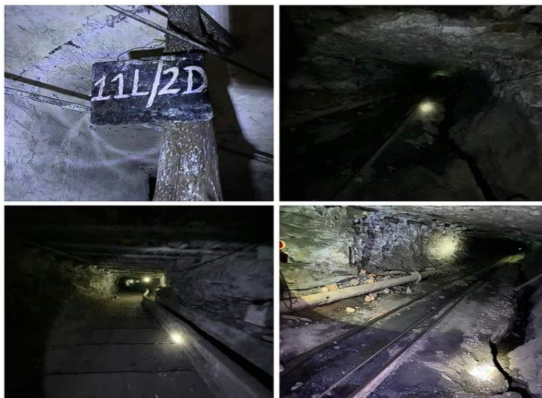
Fig. 2. The insight of Bhanora WB Colliery (U/G) mines in Bhanora (Sripur), West Bengal
